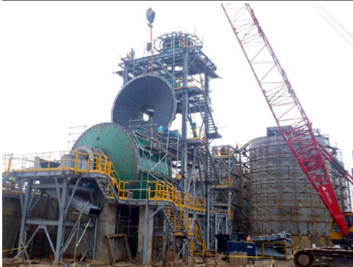
Figure 28: SAG mill installation
