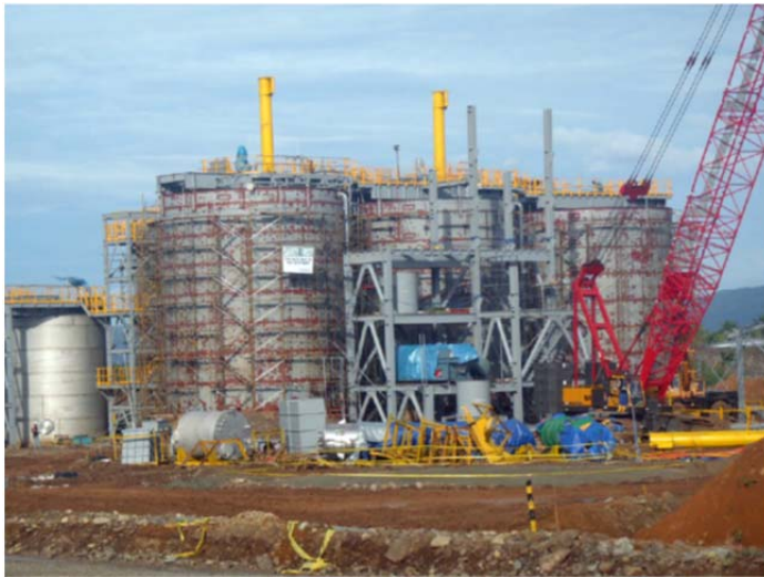
Figure 28: SAG mill installation
